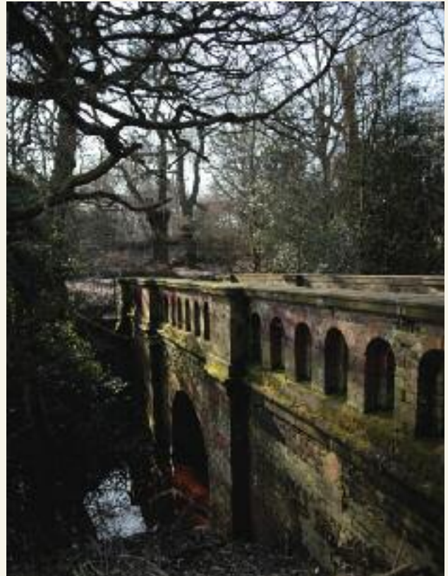
The Bird Bridge today ( Layton Thompson )
