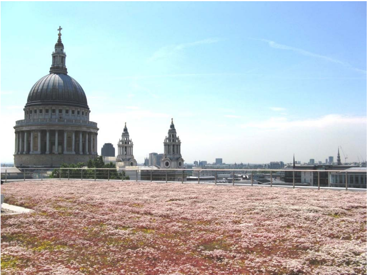
The green roof at 150 Cheapside has a spectacular view of St Pauls
